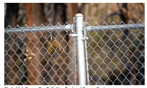
Chain Link Fence, Top Rail, Line Post and Corner Post 8900 10900 1415 955
